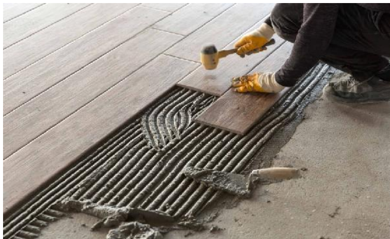
Placing of tiles with little pressure
