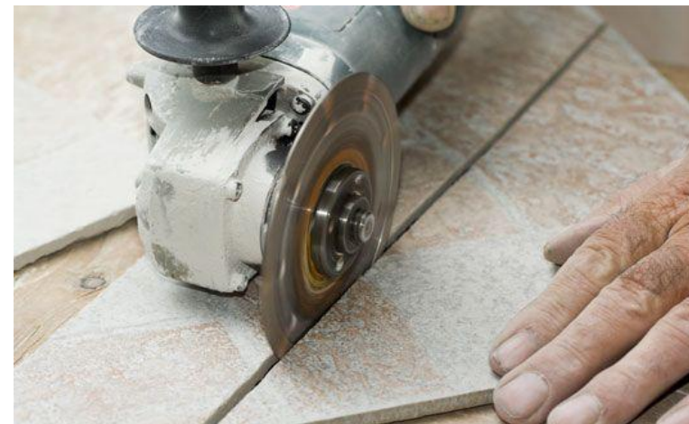
Cutting of tiles
