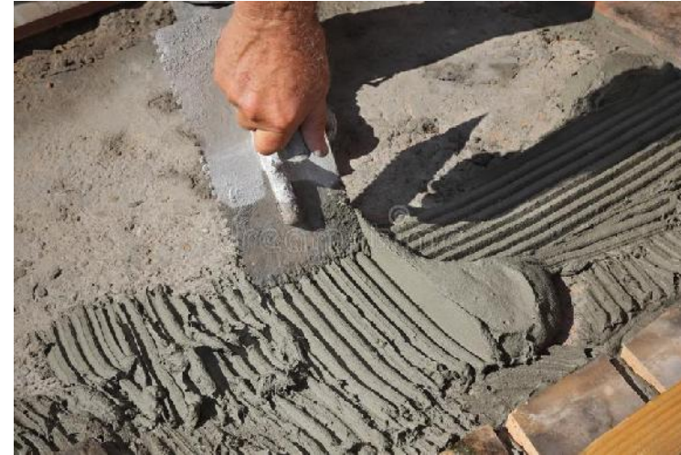
Uniform spreading of mortar with small grooving
