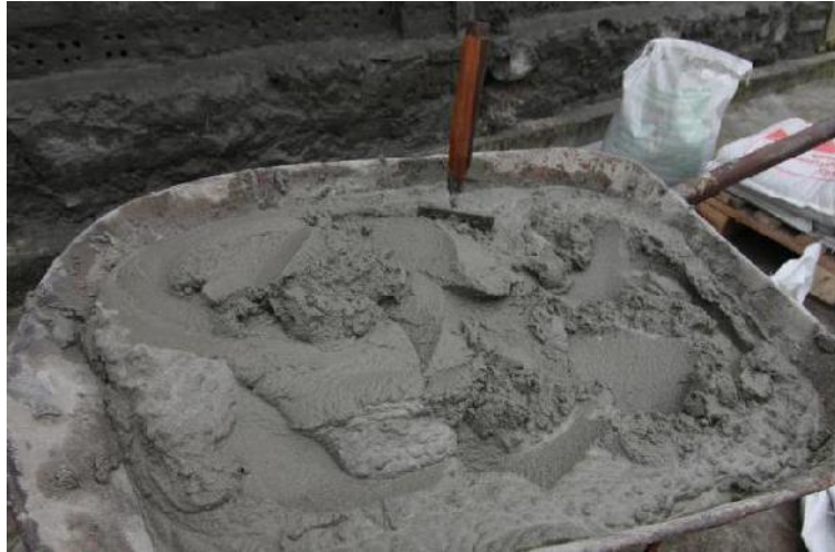
Preparation cement mortar
